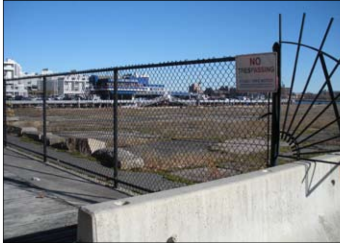
An iron fence bars public entry to the deteriorating Pier 5.
